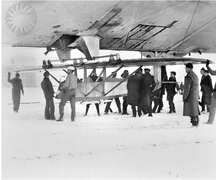
An RRG Prüfling glider attached to USS Los Angeles for carriage and drop tests.
